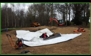
Roll out the Verde 'V' Liner, white side up so that it covers the base below. Make sure there are no creases or bumps in the grass to ensure a smooth Finish. Allow the Verde 'V' Liner to rest up the sides of the bunker, leaving a drainage channel at the top. Depending on the shape and size of the bunker, more than one piece may be required.
