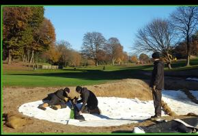
Trim the **Verde 'V' Line** artificial grass by cutting from the back side with a sharp Stanley knife and a straight edge. Try to avoid cutting across the picks where possible, to prevent fraying and ensure a neat join. Pin in place with 100m galvanised nails. If more than one piece is required, ensure the grass is pulled tight and all edges are trimmed neatly prior to making the join.
