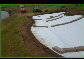
Whilst fitting the **Verde 'V' Liner**, make sure you leave a drainage channel around the perimeter. If your bunker requires a join, you can use our specialist Jointing Tape and Adhesive. Make sure the jointing tape is shiny side down, preventing water from penetrating through the tape.
