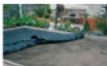
2. Lay geotextile membrane
